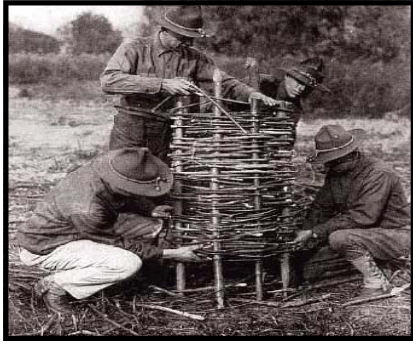
WWI trench construction
